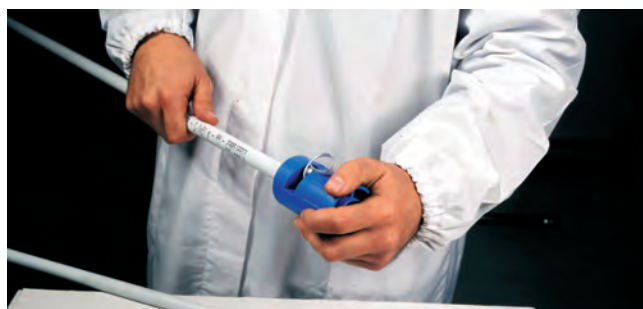
Image 23 – Dénuder le tube (steelPRES®)
