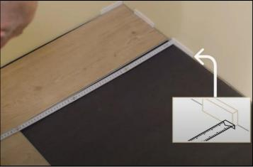
7. From the third row onwards, place the planks row by row. Make sure that you place enough spacers in the expansion joints so that the floor does not shift. Use a varying mix of decors and planks from different packs.
