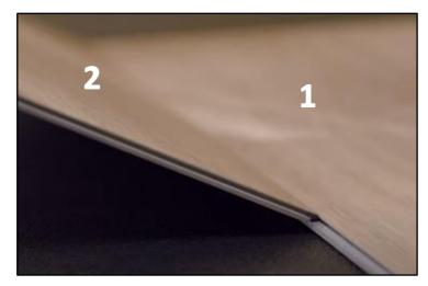
2. Now take a second plank and cut it to a minimum of 1/3 and a maximum of 2/3 of a panel length as a starting plank (n°2) for the second row.
