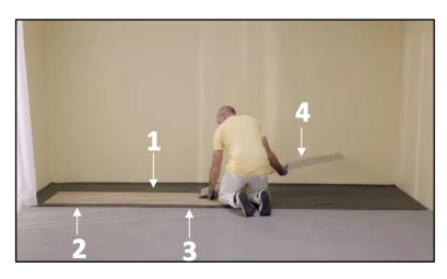
4. Place a fourth complete plank (n°4), at an angle of +30 degrees, on the long side with the tongue in the groove of the first board (n°1) of the first row and lower it. A narrow gap is now visible between board n°4 and board n°3. To do this, lift board n°4 at an angle of +30 degrees and pull it with the tongue into the groove of board n°3.
