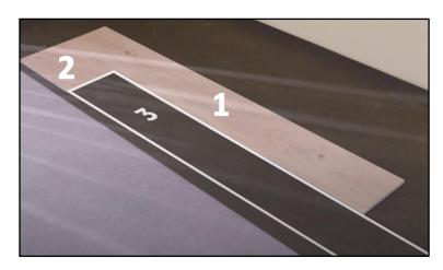
3. Take a third full length plank (n°3) of your choice. Place the board on its end with the tongue in the groove of the board (n°2) at an angle of  $\pm 30$  degrees and then lower it.
