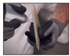
In case of a double pipe, drill a hole with the same diameter as the pipes at all the marked points, adding 15 mm. If the pipes are on the long side of the board, make a 45 degree cut from each hole to the side of the board.
