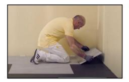
8. Place the piece of tile that is cut in the groove of the last complete tile. The first row of tiles is now complete. Once again, ensure that the tiles remain in a straight line with each other and fix the floor with sufficient spacers.
