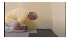
6. The last incomplete tile of the first row should now be fitted. Measure the distance from the top edge (decor) on the short side of the last full tile to a 5 mm distance block, which has been placed against the wall. Caution! Make sure that you do not start measuring from the groove, but from the top edge of the tile!
