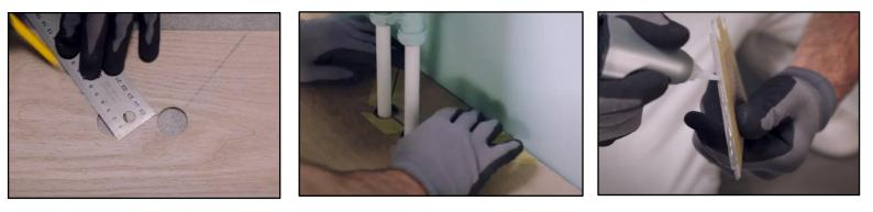
In case of a double pipe, drill a hole with the same diameter as the pipes at all the marked points, adding 15 mm. If the pipes are on the long side of the board, make a 45 degree cut from each hole to the side of the board.
