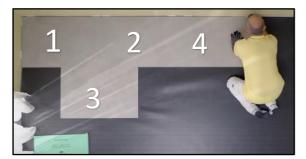
4. Take a third, complete tile (n°4) and click it into the short side of the second tile (n°2). Again make sure the tile is completely in line with the other tiles. Place a placeholder on the long side of the second (n°2) and third (n°4) tile of the first row.
