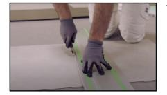
7. Draw the measured distance on a new full tile starting from the top edge (decor) on the short side where the tongue is located. Do not include the tongue. Now cut, with the aid of a ruler and a sharp Stanley knife, two or three times over the piece to be shortened. Then turn the tile with the decor side down and break off easily the cut off piece.
