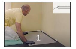
Start with a first, full length tile (n°1), which comes in the top left corner of your room. Preferably lay the 2 sides with tongue towards the walls and make sure that the expansion joint of 5 mm is respected. The groove or tongue is not part of the expansion joint. Cut them off if necessary.
