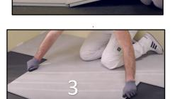
Place a tile as a "placeholder" (n°3) on the long side of the first (n°1) and the second tile (n°2). This is not the final position of this tile, but ensures that the first two tiles remain in one straight line. Check that the seams fit tightly.
