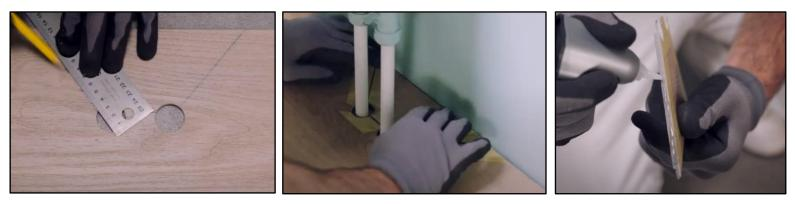
In case of a double pipe, drill a hole with the same diameter as the pipes at all the marked points, adding 15 mm. If the pipes are on the long side of the board, make a 45 degree cut from each hole to the side of the board.
