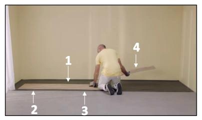
4. Place a fourth complete plank (n°4), at an angle of +30 degrees, on the long side with the tongue in the groove of the first board (n°1) of the first row and lower it. A narrow gap is now visible between board n°4 and board n°3. To do this, lift board n°4 at an angle of +30 degrees and pull it with the tongue into the groove of board n°3.
