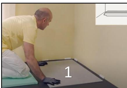
1. Start with a first, full length tile (n°1), which comes in the top left corner of your room. Preferably lay the 2 sides with tongue towards the walls and make sure that the expansion joint of 5 mm is respected. The groove or tongue is not part of the expansion joint. Cut them off if necessary.
