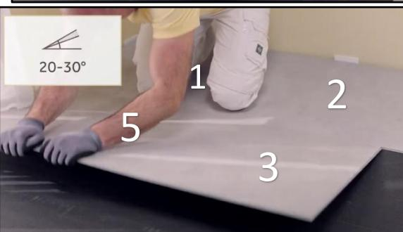
3. When a narrow gap is visible between the tiles of the first row (n°1 & 2) and those of the second row (n°3). Lift n°3 at an angle of  $\pm 30$  degrees. Keep this angle while pulling the longest side of board n°3 into the groove of board n°1. Then lower it carefully. The boards are now clicked together. If necessary, tap it with a leftover piece of tile or a tapping block
