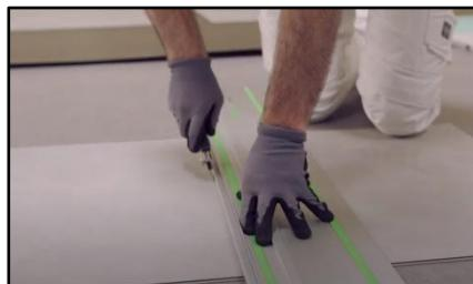
7. Draw the measured distance on a new full tile starting from the top edge (decor) on the short side where the tongue is located. Do not include the tongue. Now cut, with the aid of a ruler and a sharp Stanley knife, two or three times over the piece to be shortened. Then turn the tile with the decor side down and break off easily the cut off piece.
