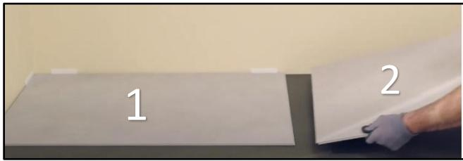
2. Take a second, full tile (n°2) and click it, at an angle of  $\pm 30$  degrees, into the short side of the first tile (n°1). Make sure that these are in a straight line with each other. Keep an angle of  $\pm 30$  degrees when installing all the tiles! This will make the installation a lot easier.
