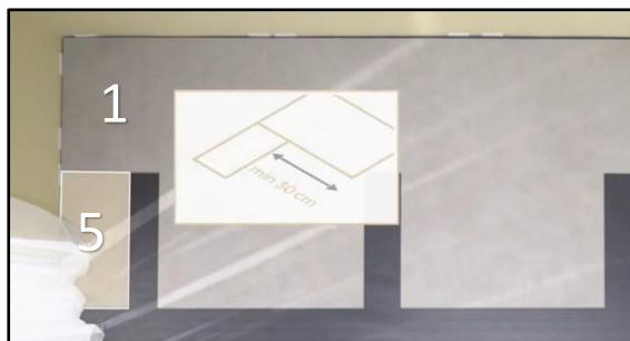
1. Take an incomplete tile (minimum 1/3 (= 30 cm) and maximum 2/3 of a tile (n°5)) as first tile for the second row. Install the tile at an angle of  $\pm 30$  degrees with the tongue in the groove of the long side of the first tile (n°1). The distance between two end joints should always be at least 30 cm. The tiles can be placed in a random pattern or in a semi-stone pattern.
