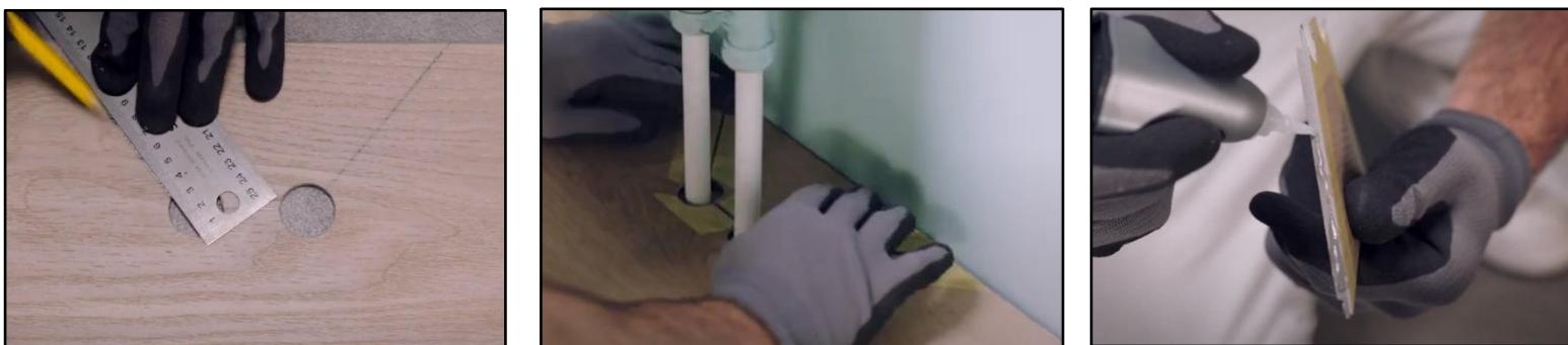
In case of a double pipe, drill a hole with the same diameter as the pipes at all the marked points, adding 15 mm. If the pipes are on the long side of the board, make a 45 degree cut from each hole to the side of the board.
