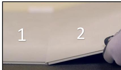
3. Place a tile as a “placeholder” (n°3) on the long side of the first (n°1) and the second tile (n°2). This is not the final position of this tile, but ensures that the first two tiles remain in one straight line. Check that the seams fit tightly.
