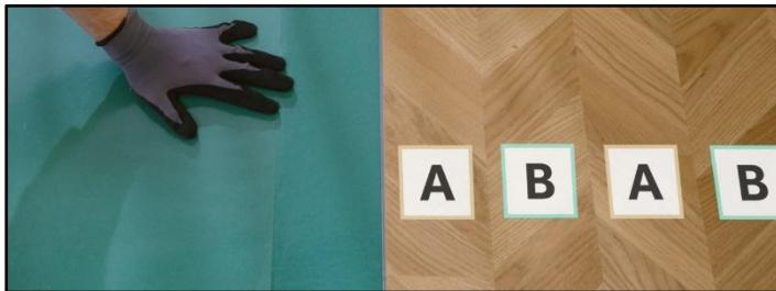
8. From the third row onwards, place the planks row by row. Make sure that you place enough spacers in the expansion joints so that the floor does not shift. Use a varying mix of decors and planks from different packs. In each row there are either all A planks, or all B planks. Each row alternates between A and B.
