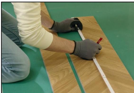
3. Measure the distance between the short edge of the second plank and the end of the first plank or the wall on the left. Take into account the 5mm expansion joint.
