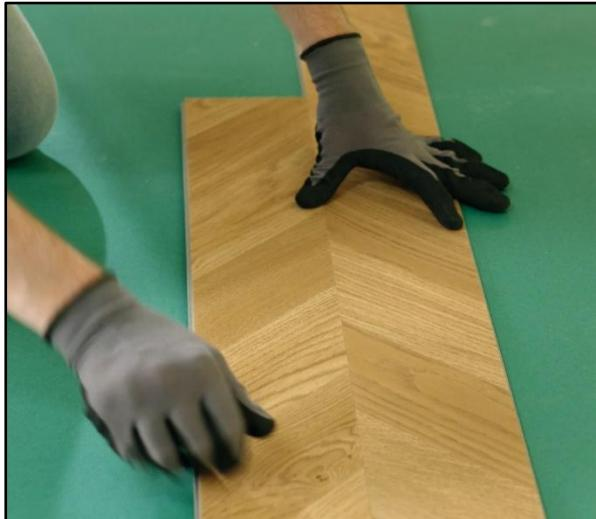
1. Start with a first, full A (or B) plank, which comes in the top left corner of your room. Preferably lay the 2 sides with tongue towards the walls, making sure to respect the expansion joint of 5 mm. The groove or tooth is not part of the expansion joint. Cut them off if necessary.
