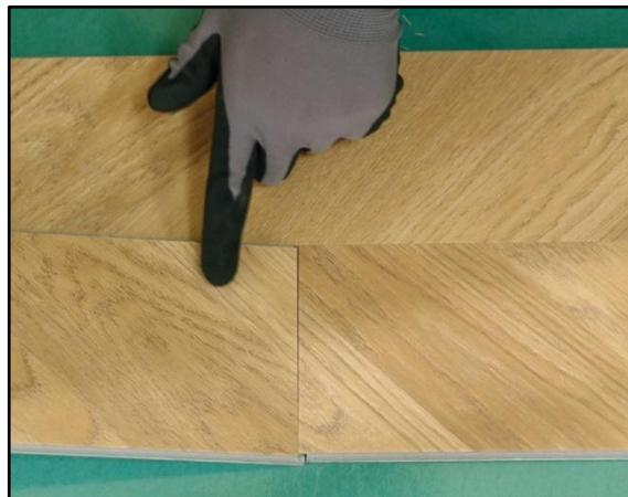
6. Place a fourth full plank A (or B), at an angle of  $+30$  degrees, on the end side with the tongue in the groove of the first plank of the first row and lower it. Now click it on the long side in the same way to the plank in the second row.
