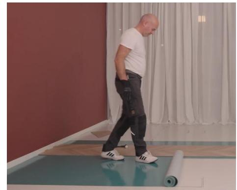
The first panel of the third row must be cut to size again. Measure the exact distance you need to make sure the pattern matches exactly. Also keep in mind that a minimum overlap of 30cm is needed with the short side of the panel of the adjacent row. Respect the 5mm expansion joint.
