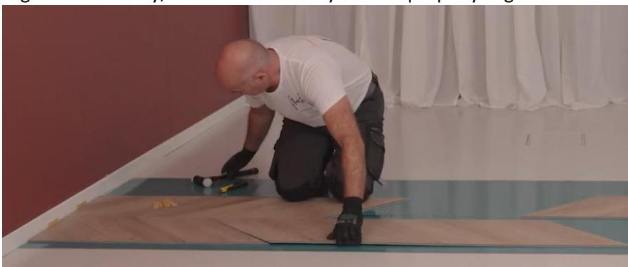
Repeat the same operation for the next panel. Work alternately with A and B panels to lay the first two rows. Always check whether the panels are properly closed.
