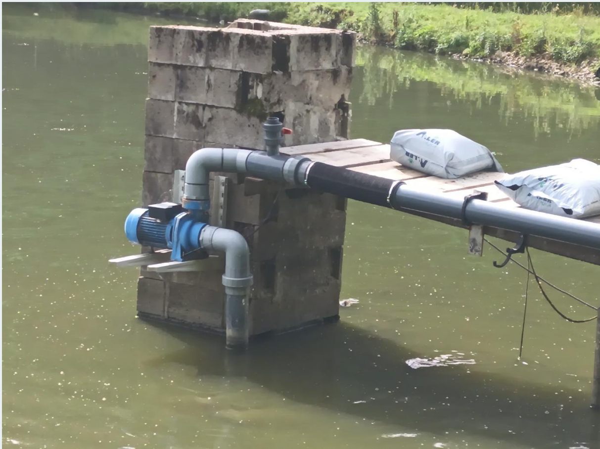
Fig. 5 Installed pump for supply of TBP system.
