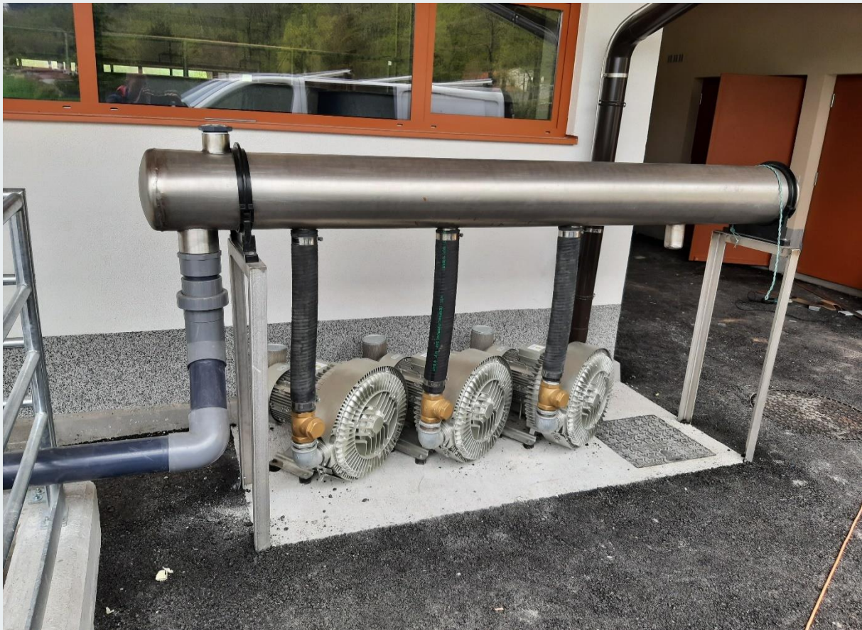
Fig. 6 Central installation of side channel blowers
