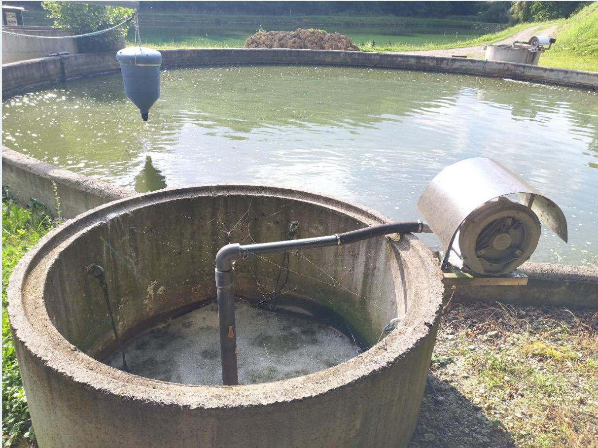
Fig. 7 Installation of side channel blowers for each airlift separately
