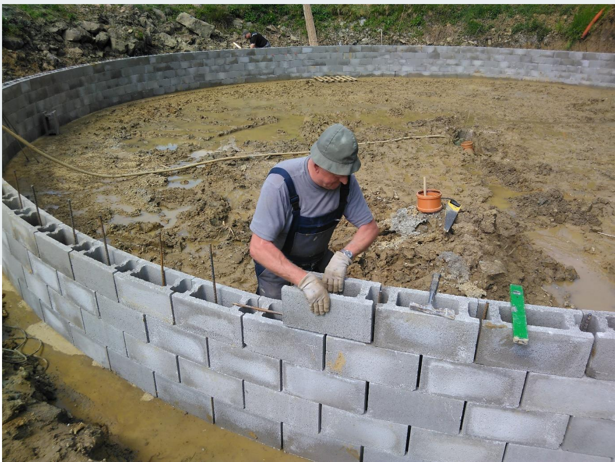
Fig. 4 TBP system during the construction.
