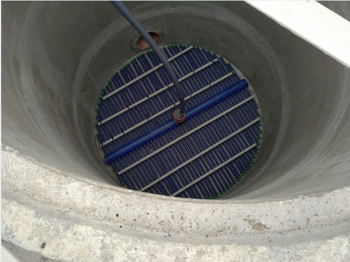
Fig. 10 Coarse bubble diffuser (pipes with drilled holes) installed in the airlift chamber
