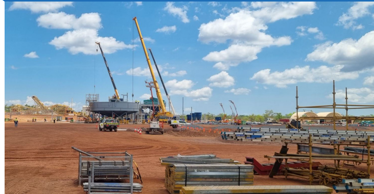
Construction work at the Finniss Lithium project site
