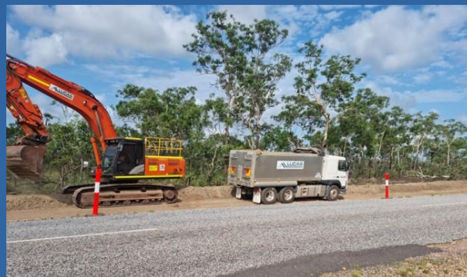
Preparations for road work at the site entrance
