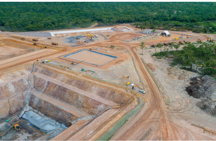
BP33 box cut December 2023.
