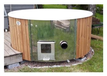
Place the hot tub on the concrete blocks and insert a roofing felt or damp-proof membrane between the blocks and wooden beams to prevent moisture migration.
