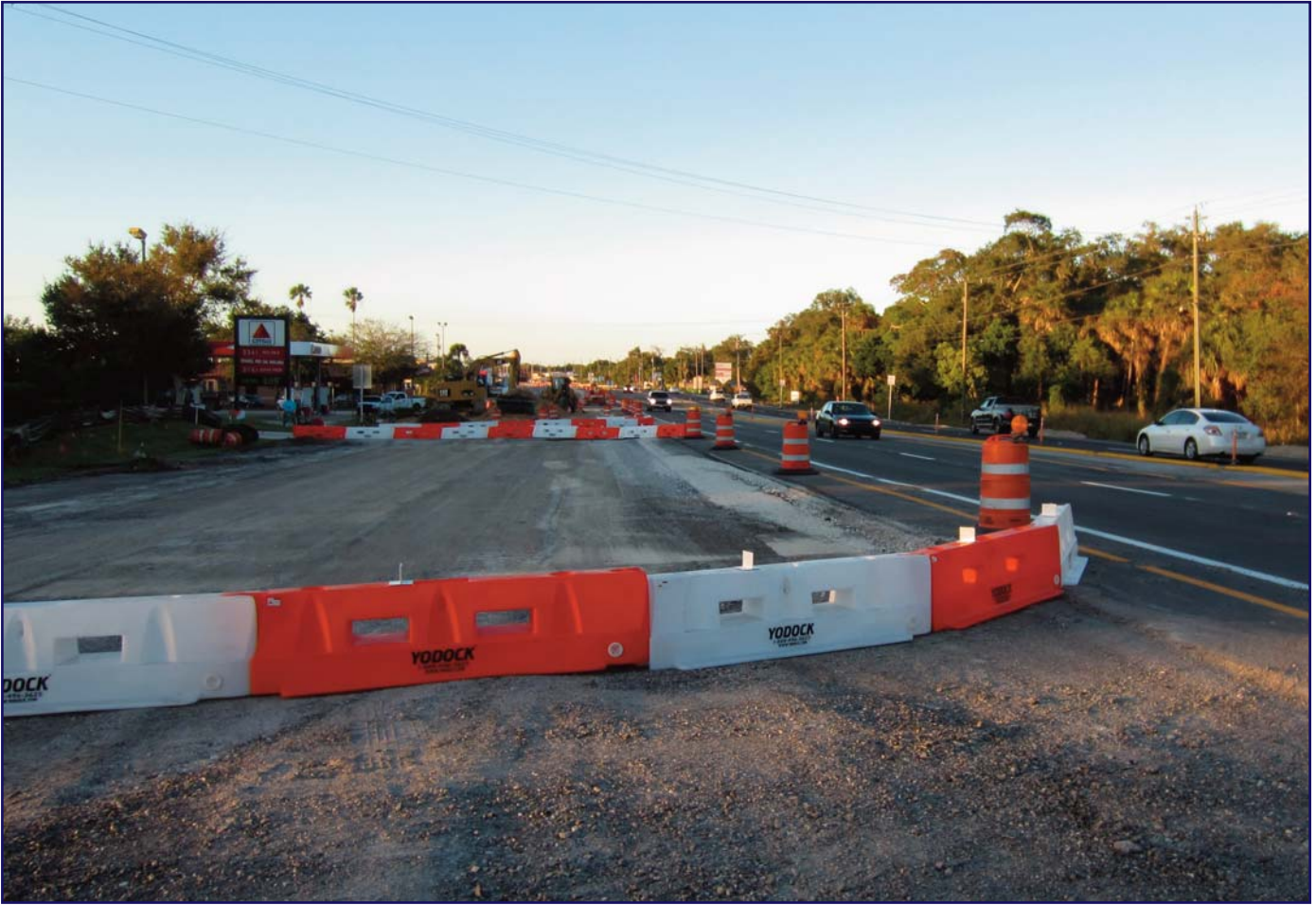
Figure 12. Use of shorter longitudinal channelizing devices to better delineate driveway access points in work zones (Source: Texas A&M Transportation Institute).
