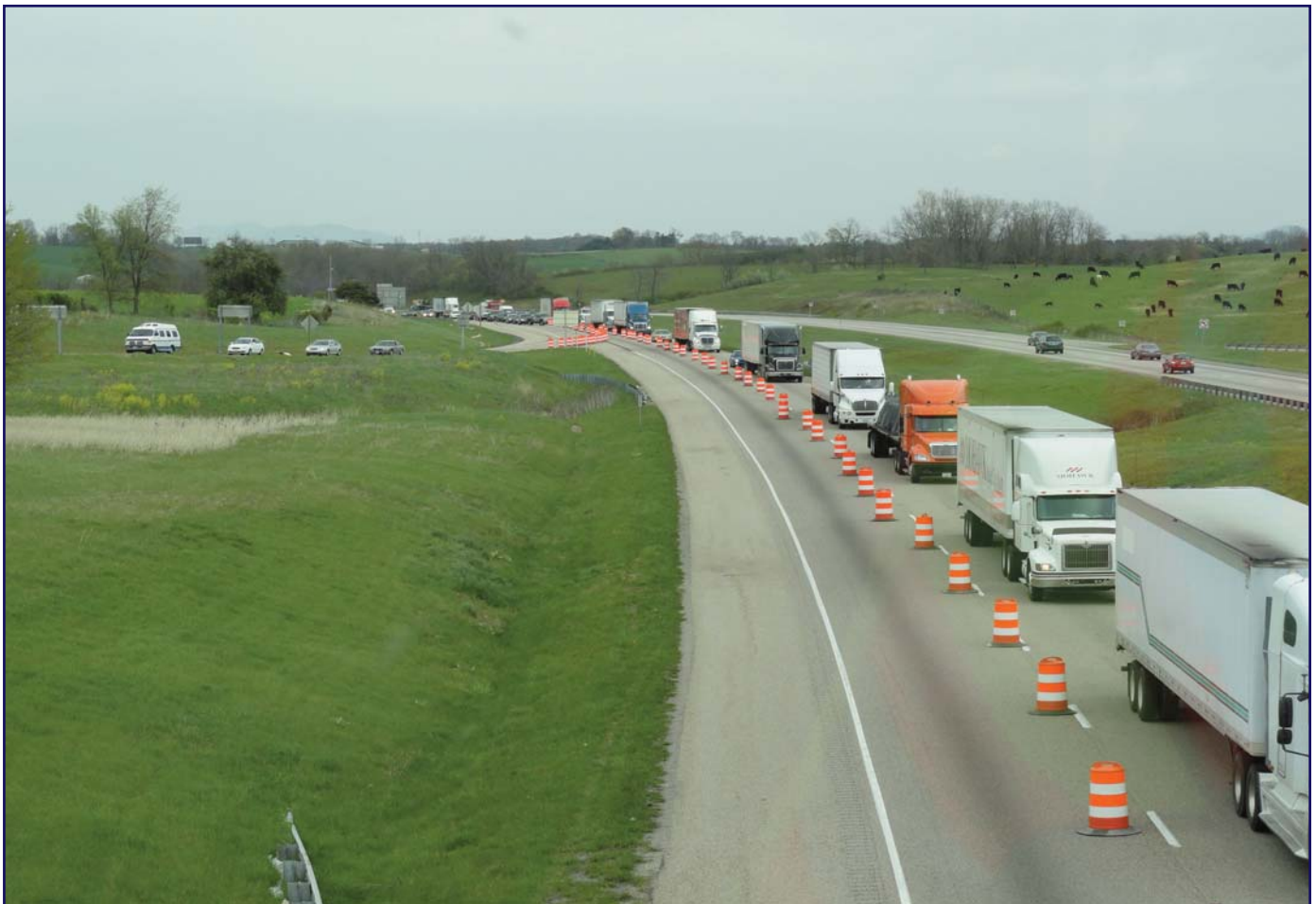
Figure 7. Creating a truck-only lane through the work zone can be an effective congestion management strategy (Source: https://farm7.staticflickr.com/6199/6124555951_9a402fe4b8_o.jpg ).
