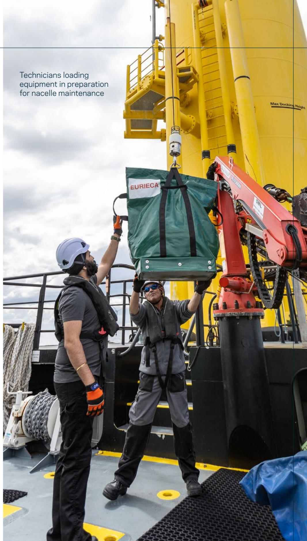
Technicians loading equipment in preparation for nacelle maintenance
