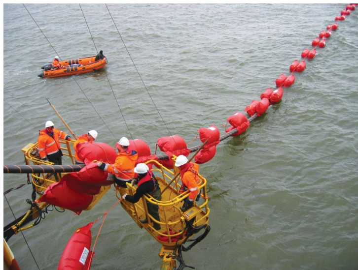
Cables being laid onto the seabed
