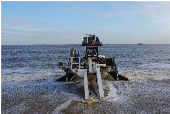
Cable laying plough on beach
