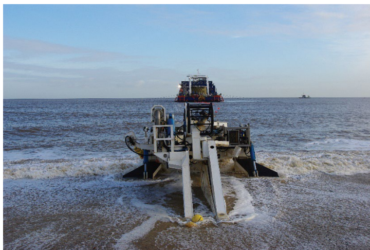
Cable laying plough on beach
