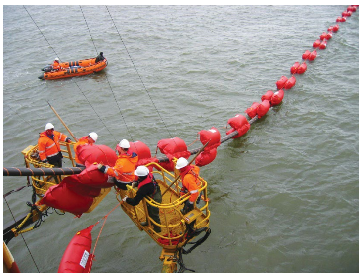
Cables being laid onto the seabed
