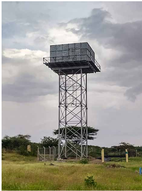
The newly constructed elevated steel tank, water kiosks, and animal watering stations on the outskirts of the Gambella Wetland. Photo: Milton Mutuma, CETRAD
