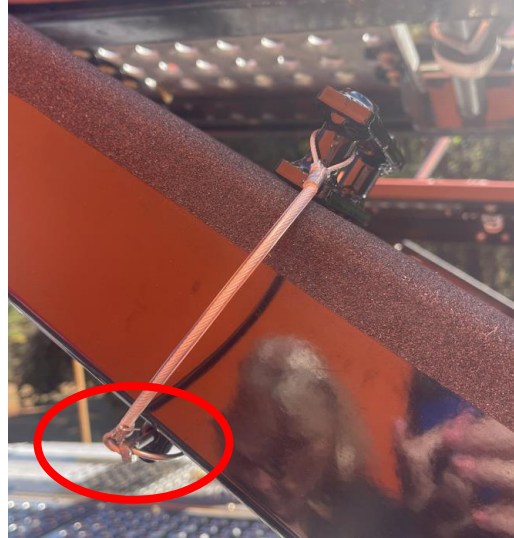
Deck Lock Pin secured with Linch Pin
