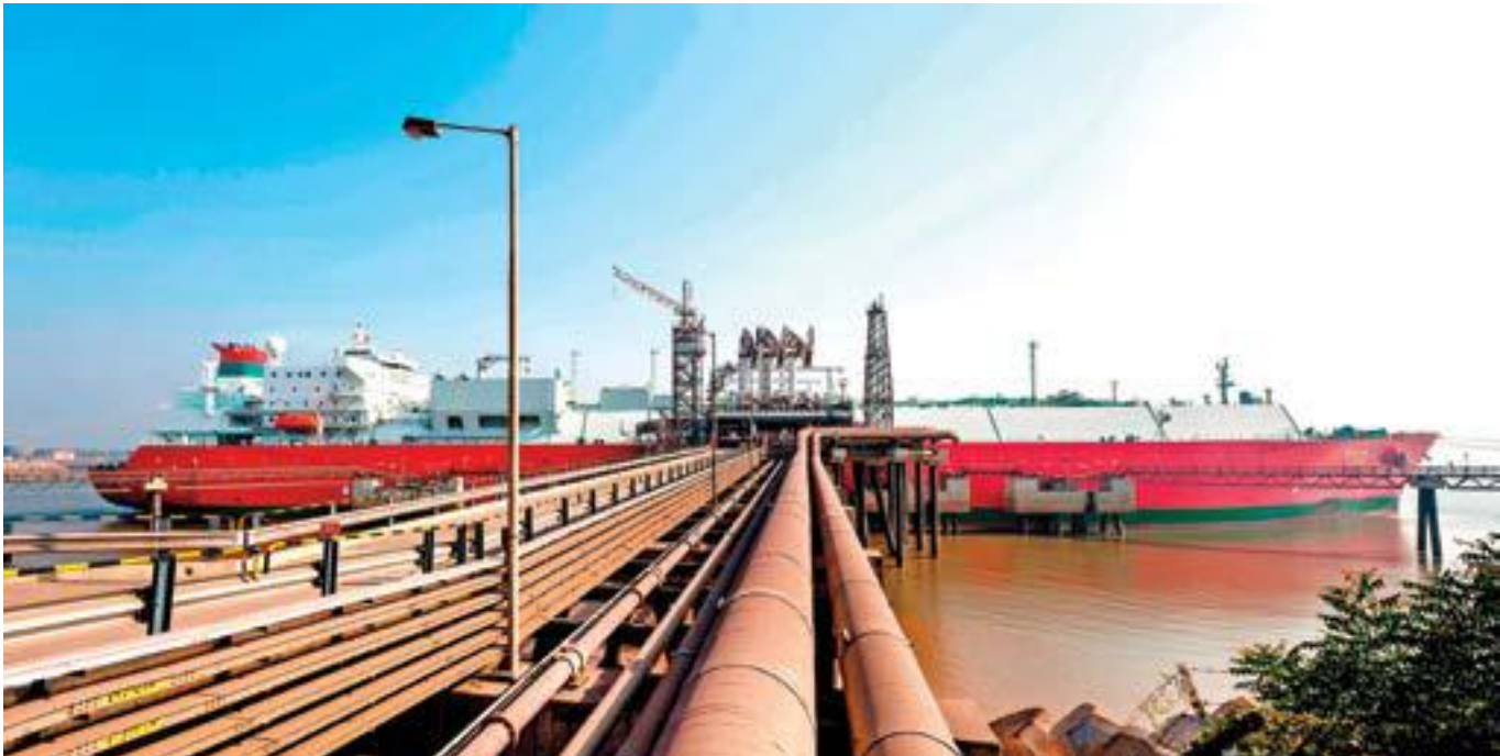
Hazira Regas Terminal - Courtesy of Shell
