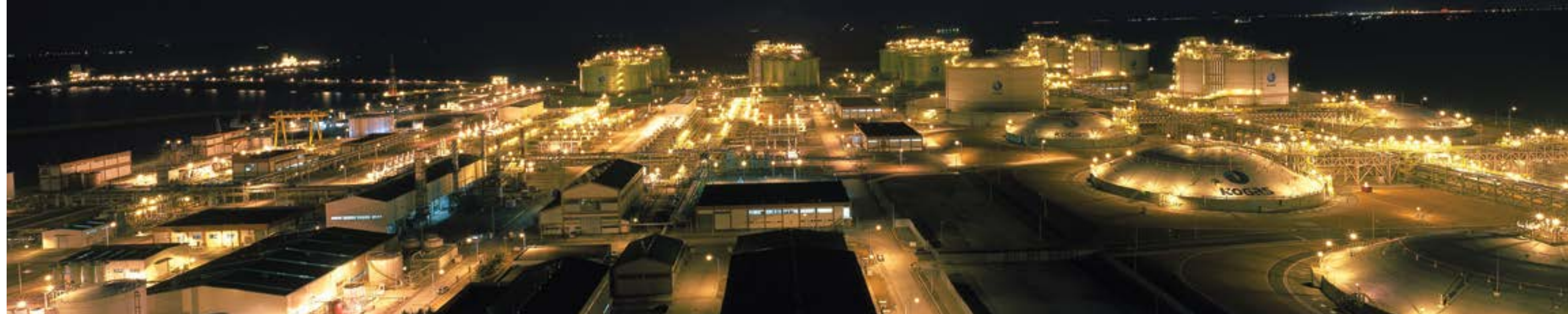
Incheon Terminal - Courtesy of KOGAS
