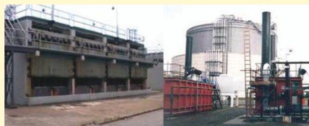
Figure 4.20 – Open Rack and Submerged Combustion Vaporisers.
