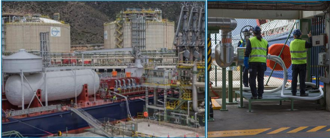
Figure 27: Bunkering facilities at Cartagena. Photo courtesy of Enagas.
