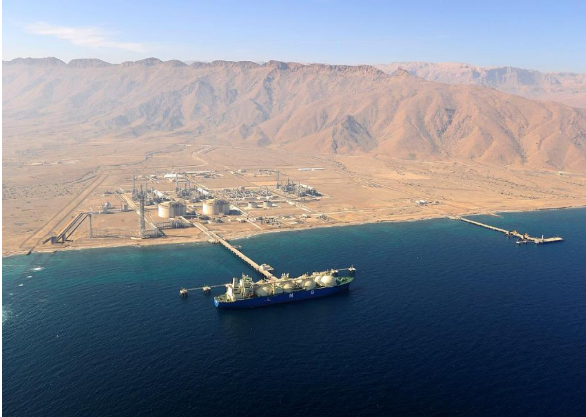
Figure 19: Oman LNG has recently undertaken modifications to process a wider range of feed gas compositions in light of new upstream developments. Photo courtesy of Shell and Khalil
