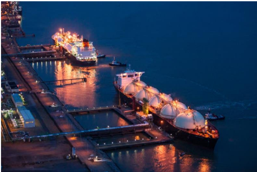
Figure 14: View of "Ben Badis" and "Gemini" LNG tankers during first LNG transshipment between two LNG tankers at Montoir-de-Bretagne LNG terminal the 7th of August 2013, France, Elengy, Engie Group – Photo courtesy of ENGIE / BESTIMAGE / WERDEFROY YANN
