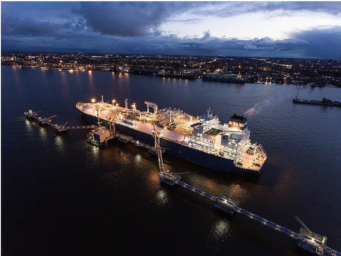
Figure 21: The FSRU Independence was delivered in 2014 to diversify Lithuania's gas imports. Photo courtesy of AB Klaipėdos Nafta at Wikimedia Commons
