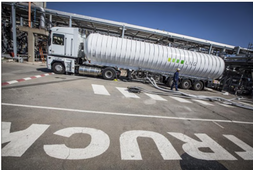
Figure 23: Two truck loading bays at Fos-Tonkin LNG terminal: End September 2014, first commercial truck loading. Photo provided courtesy of ENGIE / NEUS / BRUNET ARNAUD
