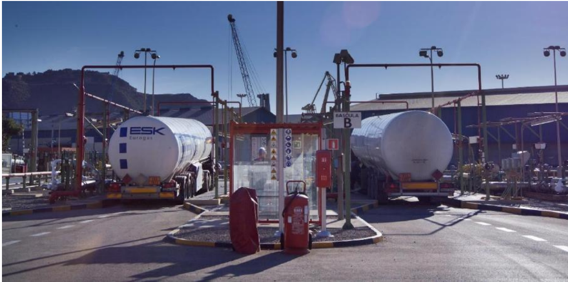
Figure 8: Truck loading stations in Cartagena Plant. Photo courtesy of Enagas
