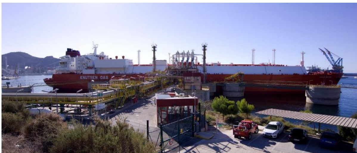
Figure 9: The Sevilla Knutsen at the Cartena Terminal. Photo courtesy of Enagas
