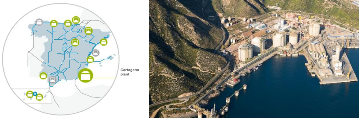
Figure 26: The Cartagena LNG Import Terminal in southern Spain has added several additional functionalities to adapt to changing market conditions. Photo courtesy of Enagas
