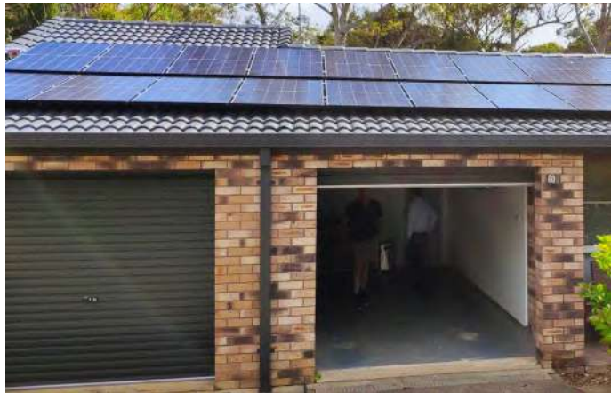
Australia, Melbourne 6kW, Growatt SPH6000
