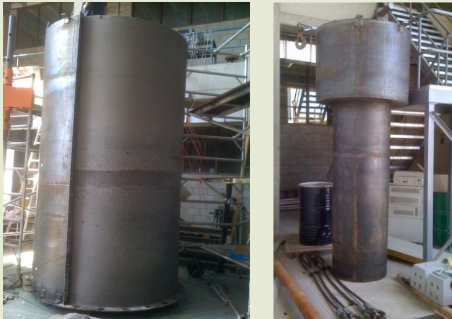
Figure 60 – Components of the first supercontainer half-scale test, which aimed to demonstrate the feasibility of fabricating the pre-cast concrete buffer component of the supercontainer, and the impact of inserting a hot overpack on this component. Left: Removal of the mould after casting the concrete buffer. Right: The inner formwork of the mould.
