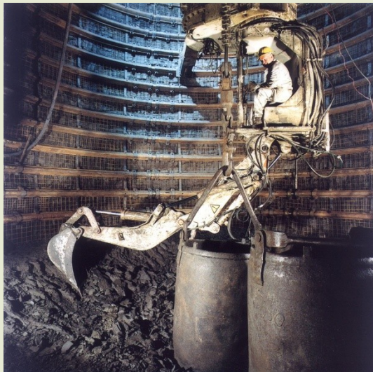
Constructing the second shaft
