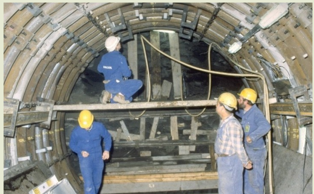
Fitting the lining at the end of the second gallery, called "Test Drift"
