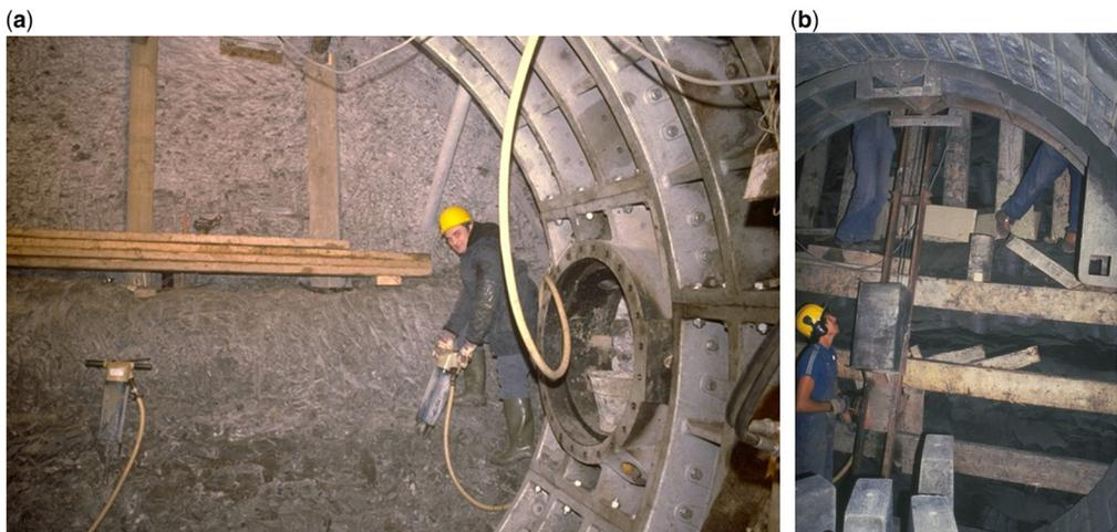
**Fig. 2.** (a) Construction of the first gallery lined with cast-iron segments. (b) Photograph taken during the construction of the Test Drift with semi-manual techniques. Each ring is composed of 64 concrete blocks (60 cm thick) with wooden plates between the segments. Source: ©EIG EURIDICE.
