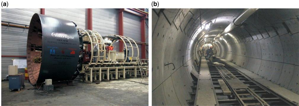
**Fig. 3.** (a) Tunnel boring machine equipped with a shield and a road header. (b) Connecting Gallery during its construction. Each ring is composed of 10 segments (40 cm thick) and two counter key segments (Bastiaens *et al.* 2003).
