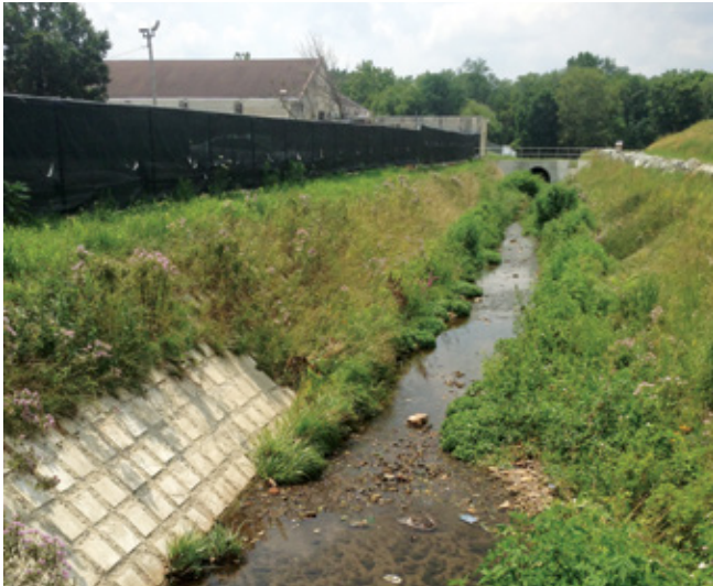
Figure 10. Stream inside the remediated asbestos waste site in Ambler, PA.
