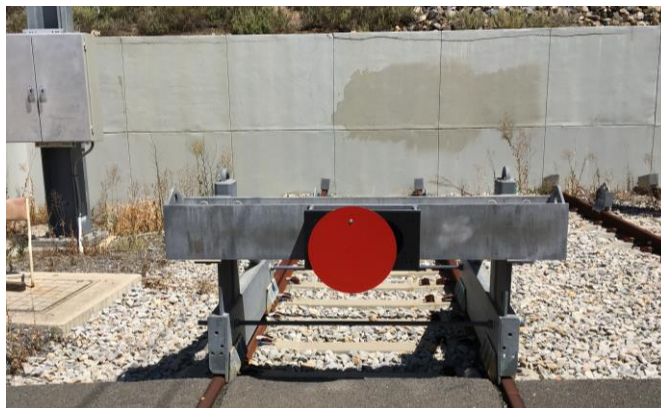
Figure 1: Friction buffer stop
