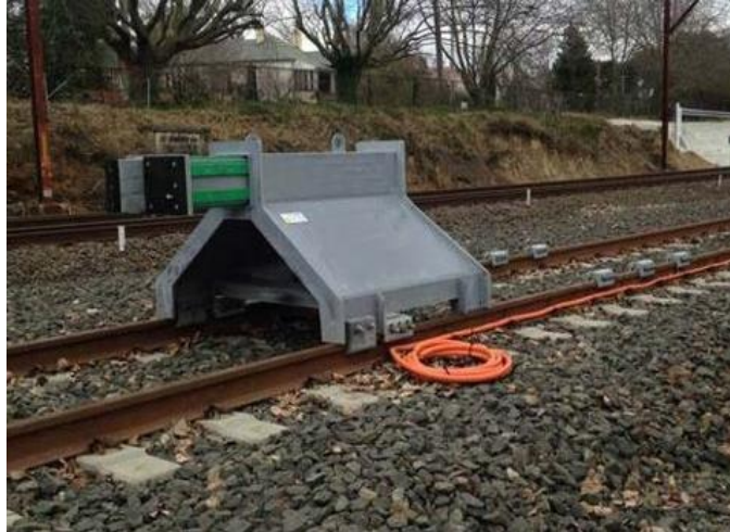
Figure 3: Combination of friction and hydraulic buffer stop
