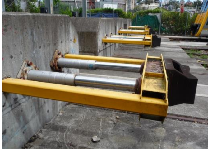
Figure 2: Hydraulic buffer stop
