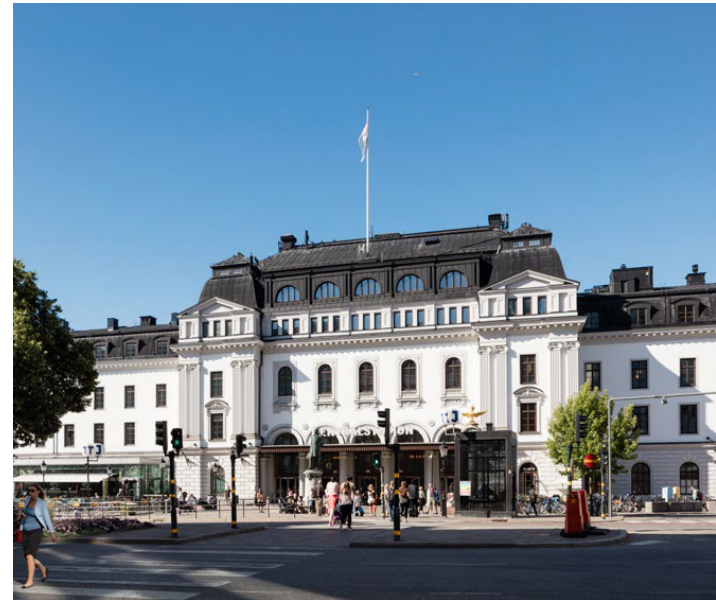
STOCKHOLMS CENTRALSTATION BRAND CENTRAL STATION
