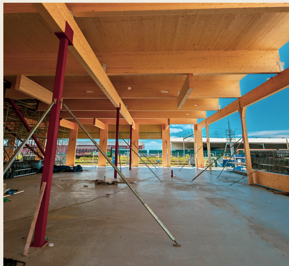
The wooden frame is assembled by KL Projekt AB. Photo: KL Projekt AB
