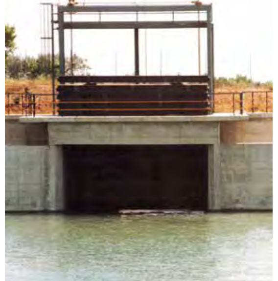
On-Off Penstock for basin 2500x2500 mm Welded Carbon steel
