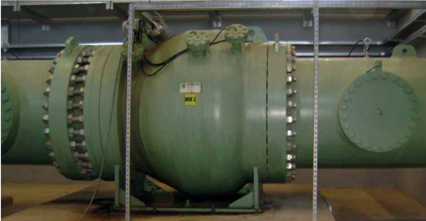
Non-return axial valve DN 1400 ASME/ANSI 600 Algeria
