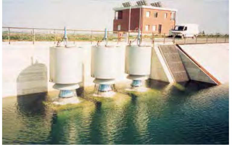
▼ Capitanata Plant (Italy) Tank level control valves
