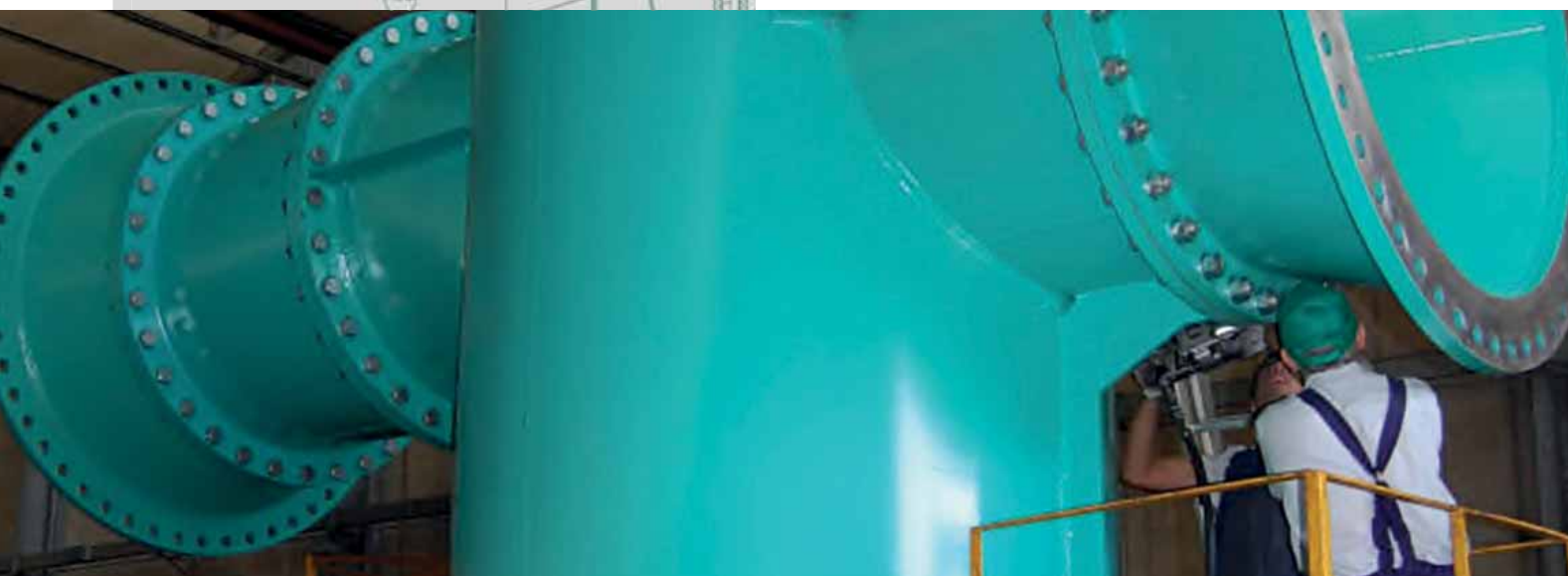
Double flanged sleeve valve DN 1500 PN 10 Saudi Arabia
