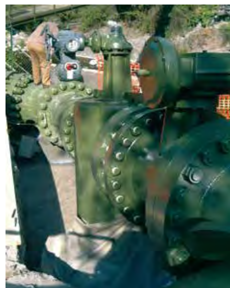
Double flanged sleeve valve ▼ DN 600 ANSI 600
