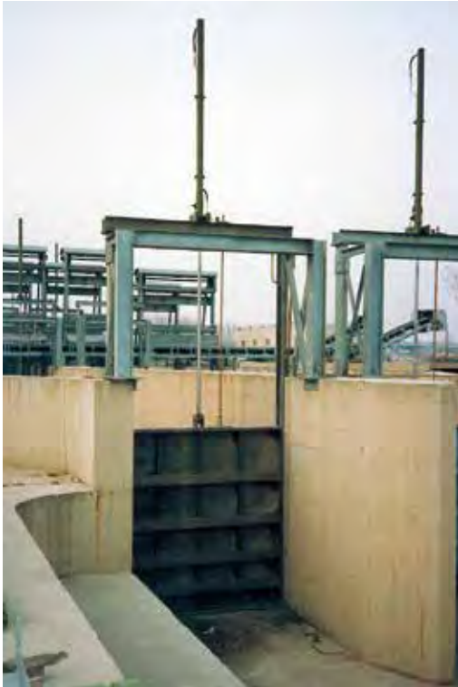
Penstock - 2000x2000 mm Welded carbon steel
