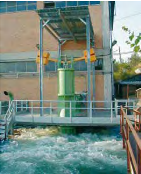
► High Pressure Control Valve DN 400 PN 25 Welded carbon steel
