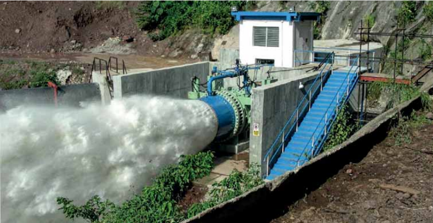
Butterfly valve DN 2000 PN 16 Under exceptional discharge condition - Venezuela
