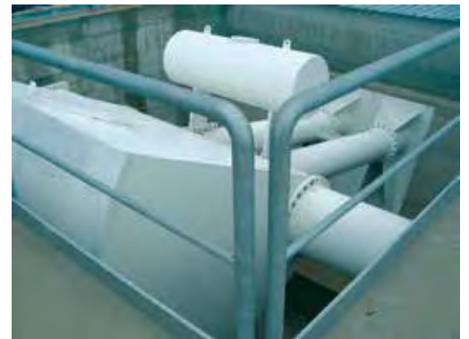
High Pressure Outlet Slide Gate 3000x3000 mm Head 45 m.w.c. Welded carbon steel
