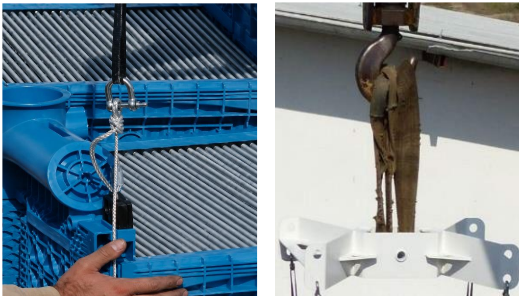
Figure 9: Fixing lifting arrangement
