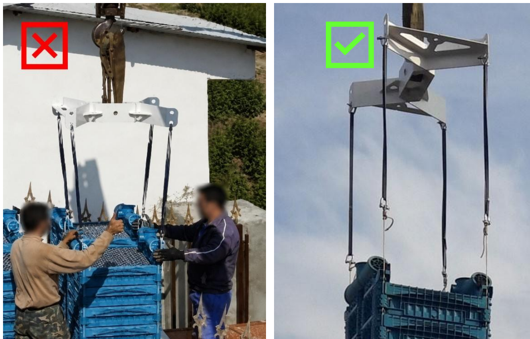
Figure 10: Lifting a tower with the Lifting Tool
