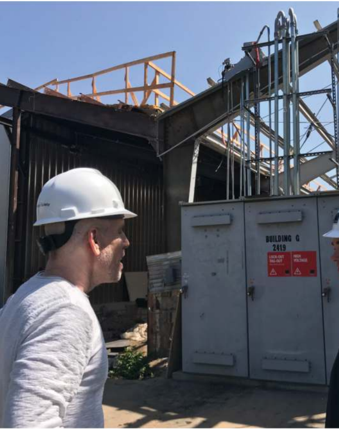
Figure 3: Michael Knopoff gives us a tour of the construction site at Bergamot Station
