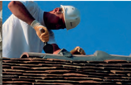
MASONRY OF TILES
