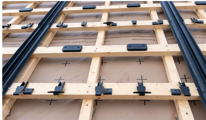
Substructure of the 3S Alpine+ solution: five Alpine hooks and in this case two rubber supports allow the 3S solar roof to be used in high Alpine regions.
