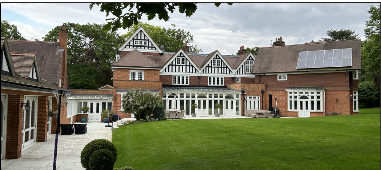
View of rear of manor house, rear extension, and side annex
