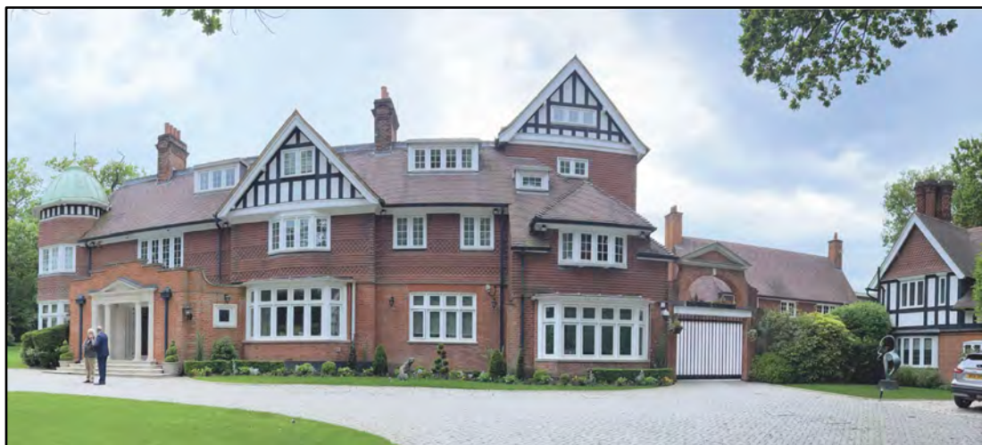
View of front of existing Manor House, gate house and annexe
