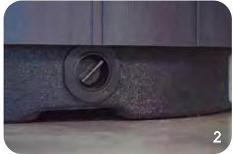
Locate the drain valve at the bottom end of the spa cabinet.
