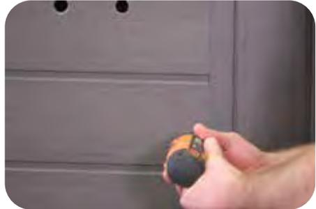
Push the SmartLink™ connector cable through one of the holes.
