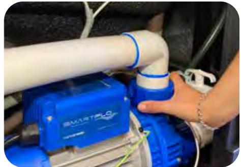
Only tighten the barrel union by hand
