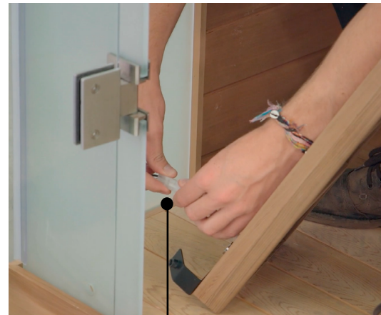
Attach front panel power cable to sauna base cable
