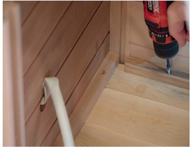
Screw long piece along back side wall
