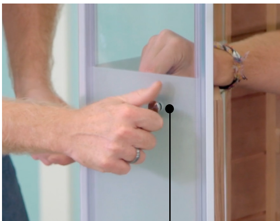
Insert screws into the glass panel through the front heater bracket
