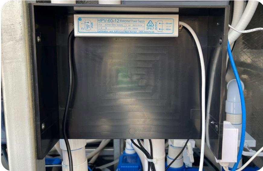
**Step 5:** Using four small screws attach SmartStream™ box to the black box.
