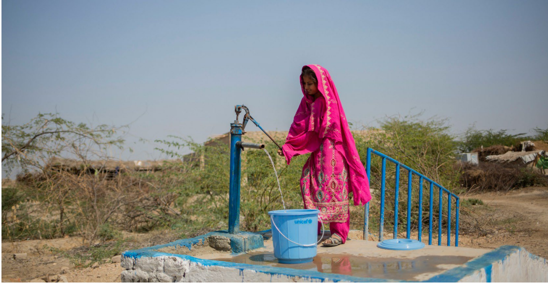
Farzana, 12, pumps clean drinking water from a UNICEF-installed, climate-resilient hand pump located just 5 minutes from her home in Umerkot district, Sindh Province.
