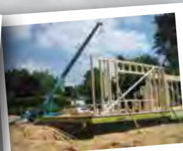
Timber Frame Work
