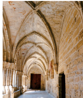
A groined cross-vault.
