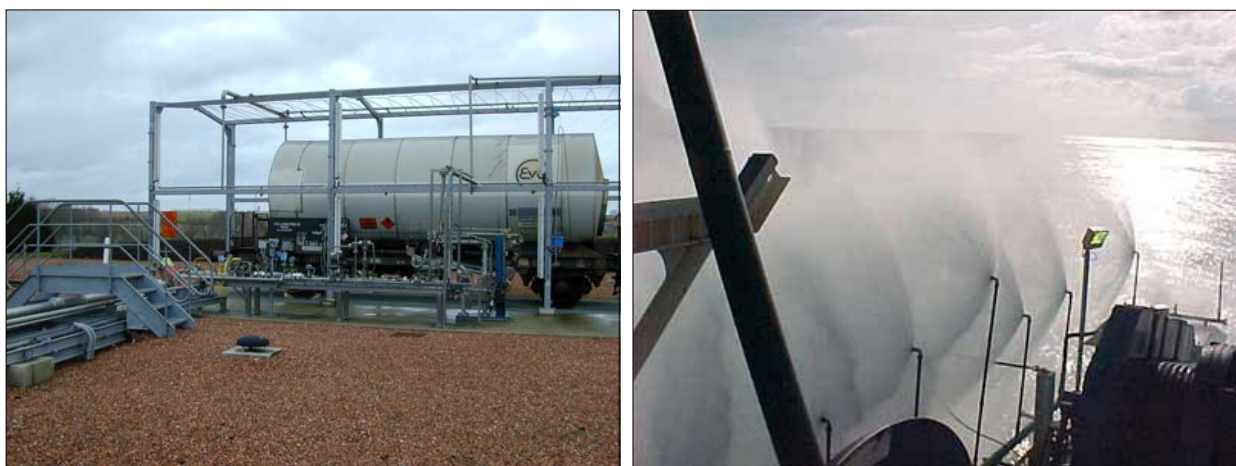
Figuur 5-1 Ketelwagen losstation (bron: TNO) en offshore platform (bron: www.rigcooling.com).
