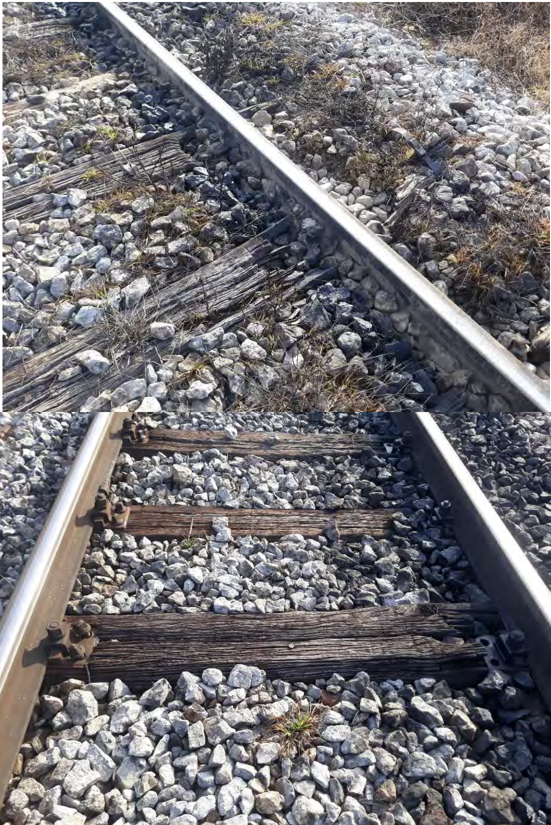
Figure 4.2.6.1: Appearance of the wooden sleepers in the serious accident zone (source: “IŽS”a.d.)
