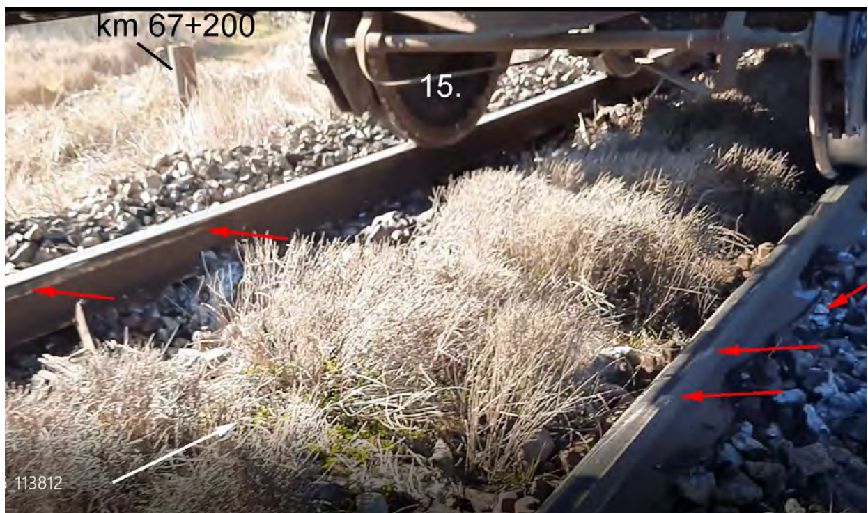
Figure 4.2.1.17: Trace of derailment on the right rail
