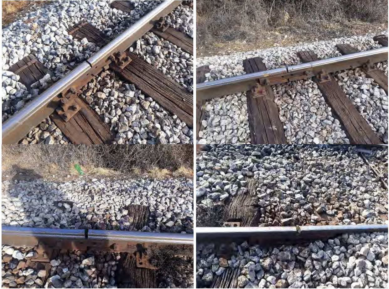
Figure 4.2.9.7: The appearance of railway joints in the broader area of the serious accident (floating unbalanced joints)
