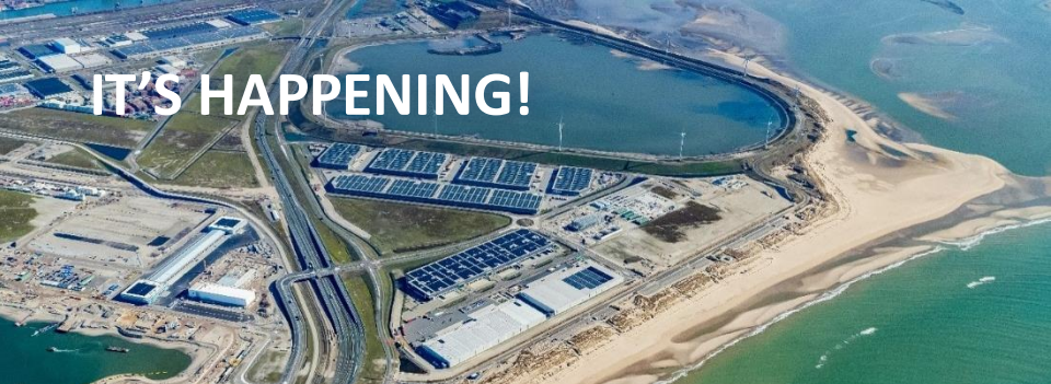
Building site Conversion park
