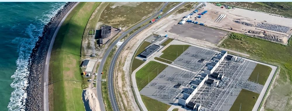
Offshore wind landfall
