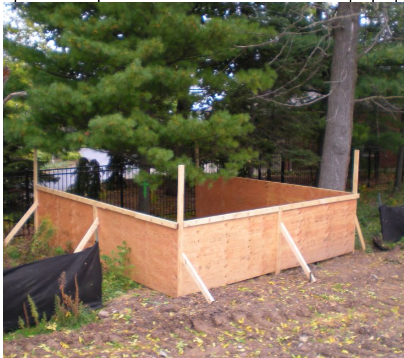
Example of a tree protection barrier for a tree on private property
