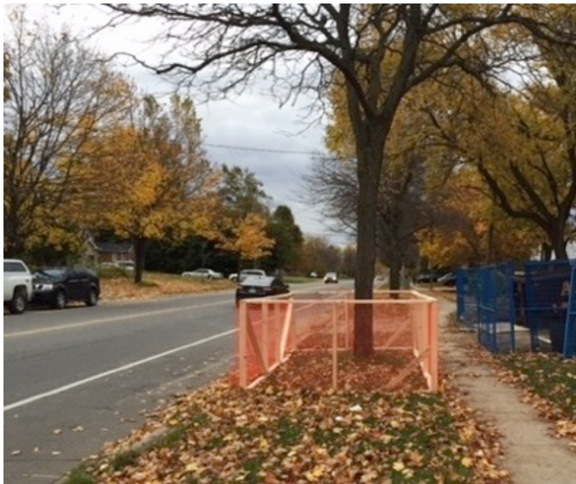
Example of a tree protection barrier for a tree on municipal property.
