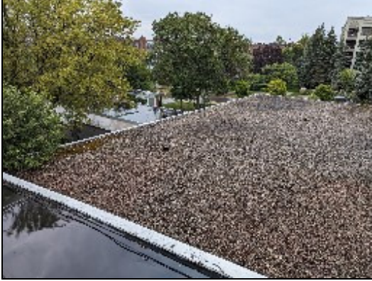
9. Flat roof - BLDG-4
