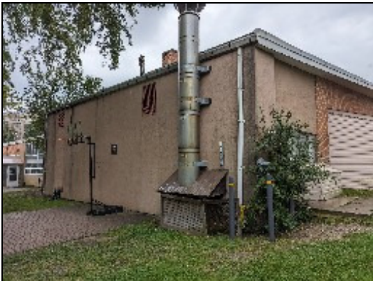
7. Two downspouts for BLDG-3
