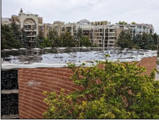
15. Flat roof - BLDG-5
