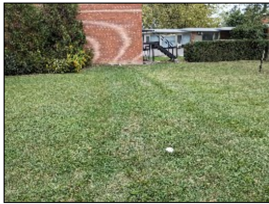
6. Combined sewer lateral (cleanouts) CO-COMB-1 on grass
