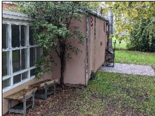
8. Two downspouts for BLDG-3
