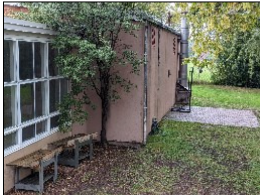
8. Two downspouts for BLDG-3
