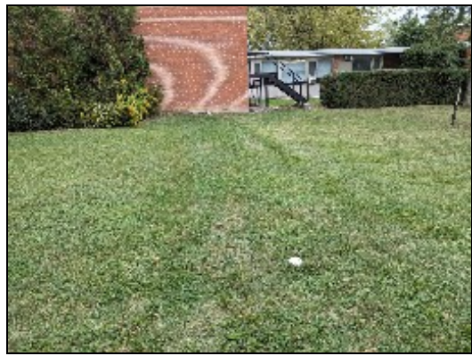
6. Combined sewer lateral (cleanouts) CO-COMB-1 on grass
