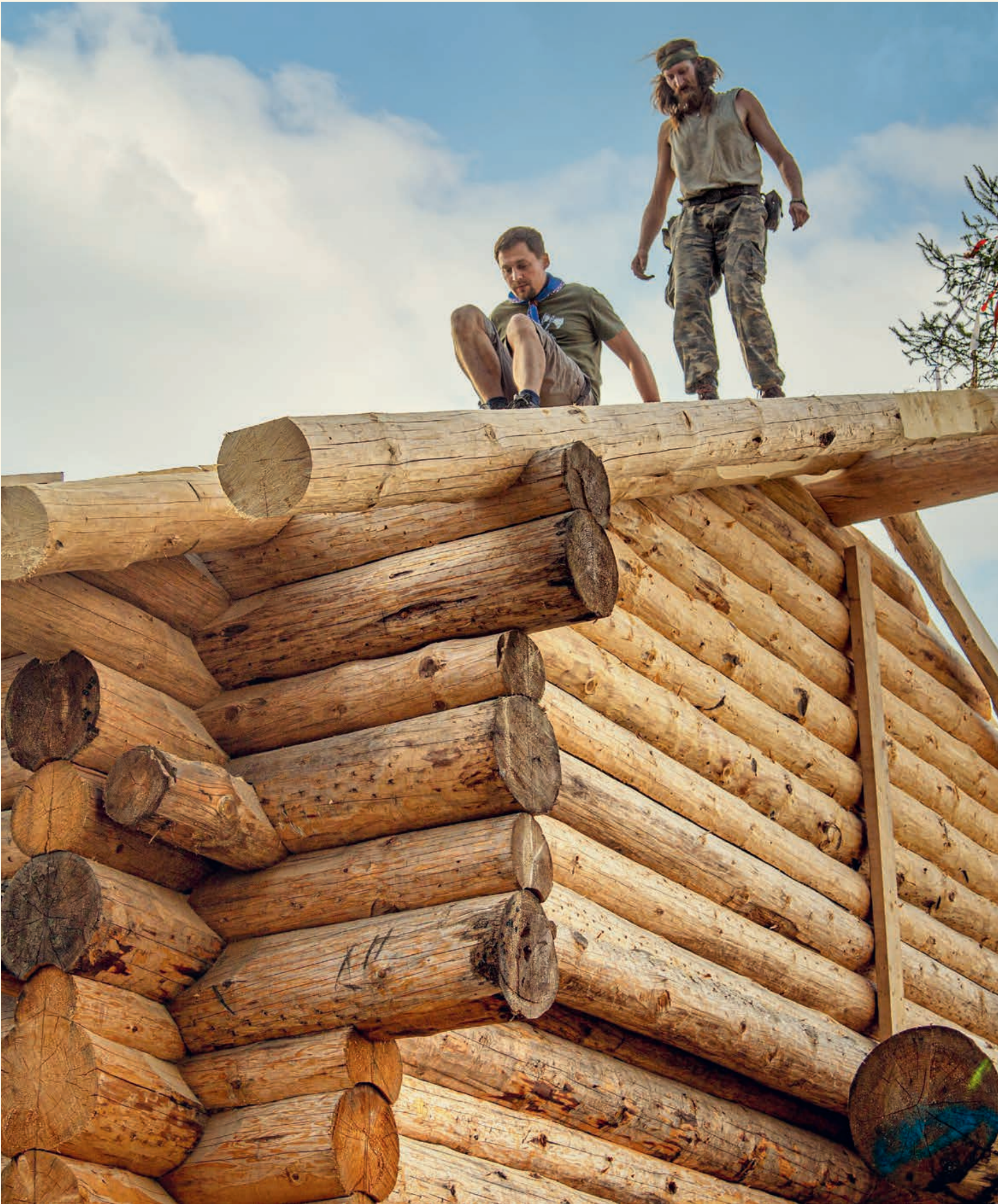
Construction of the Ostrá Hürka Háj scout hut, Silesia.
