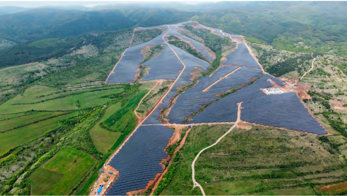
Bulgaria's largest solar power plant, Verila, supplying electricity to CETIN and Yettel
